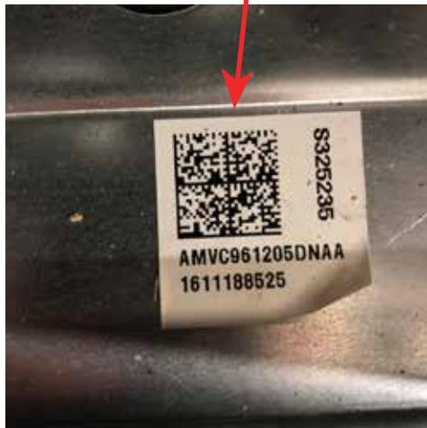
For this **ComfortNet** furnace, the 2D barcode is located on the blowerdeck, its model number is AMVC961205DNAA
